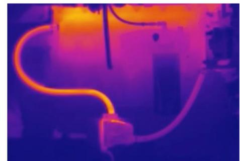
*Thermosiphon Heater Hot Spots, Boiling Temperature*
